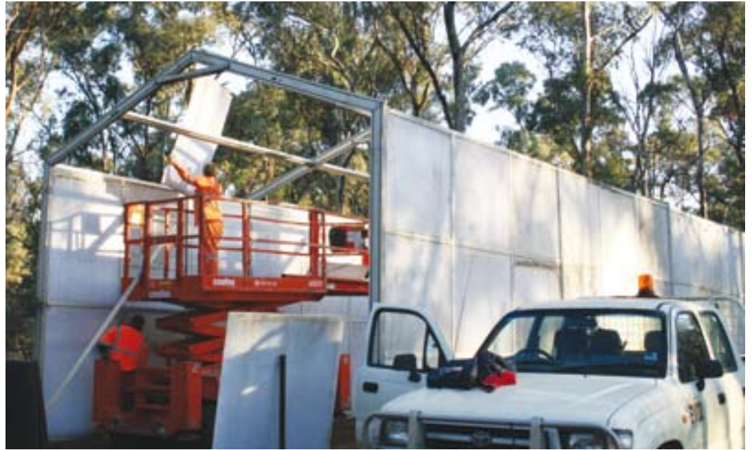
Erecting the shed for the drill rig at Eaglehawk North.
