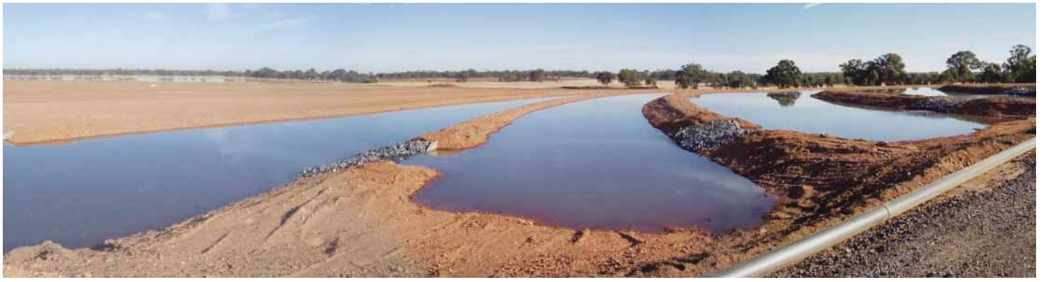
Above: the new pond at Woodvale has a tiered design to maximise the evaporation area.
