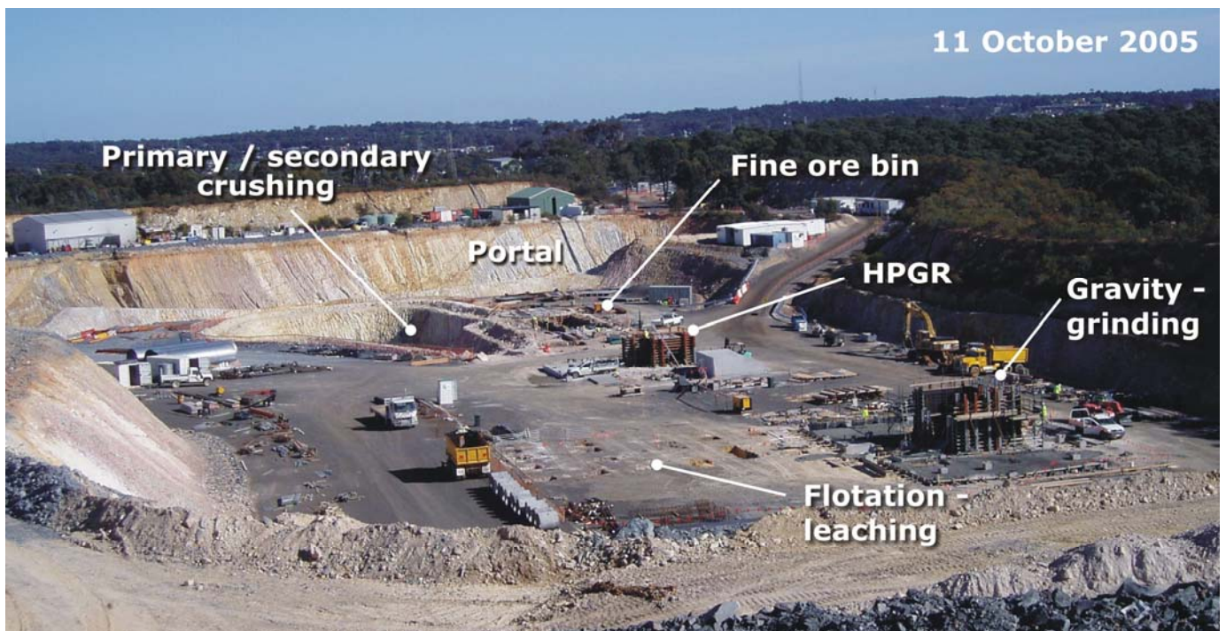
South mine gold plant construction: Carshalton Site.
